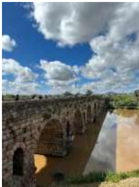
Figure 5: Bridge over the Guadalquivir
