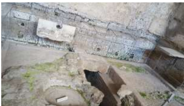
Figure 11: Crypta Balbi's exedra's toilets
