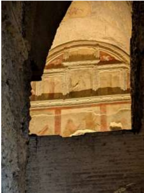
Figure 6: The stucco wall within the Domus Tiberiana rooms
