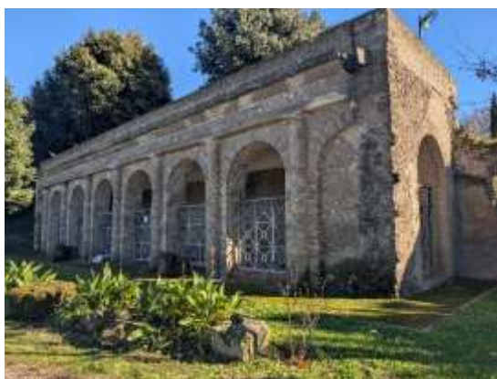
Figure 26: The portico of the Sanctuary of Juno Sospita
